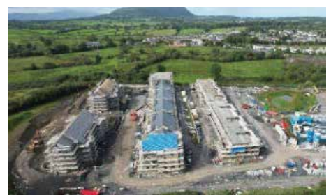
Maugheraboy Development in construction
