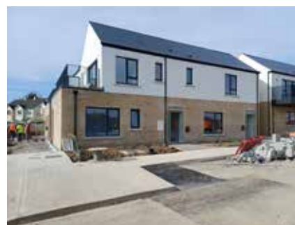
Phase 1 Nearing Completion at Camross
